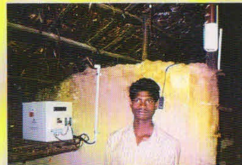
HLS Installation- An inside view
