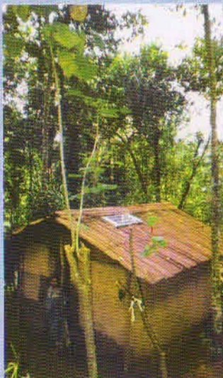
A typical HLS installation, deep inside the forest
