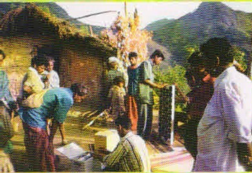
Preparing for Solar Home Lighting System Installation
